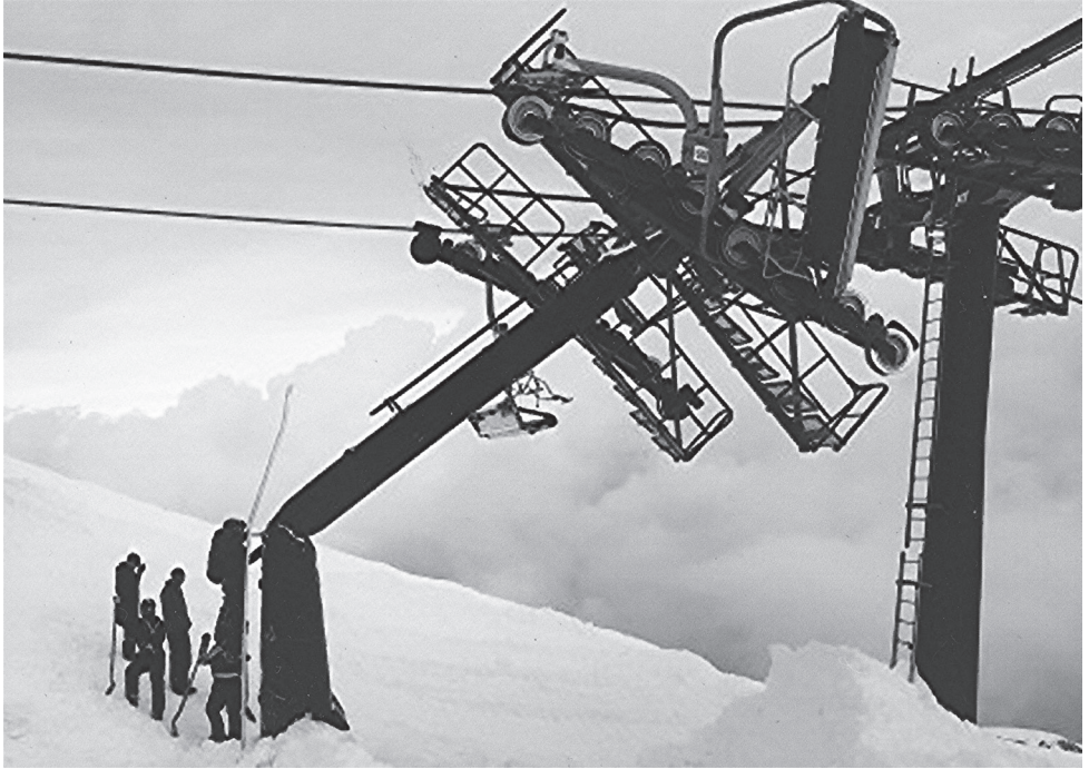
The top tower on the High Noon Express six-seater chairlift at Turoa after it was hit by an avalanche in August. Photo: RAL.
